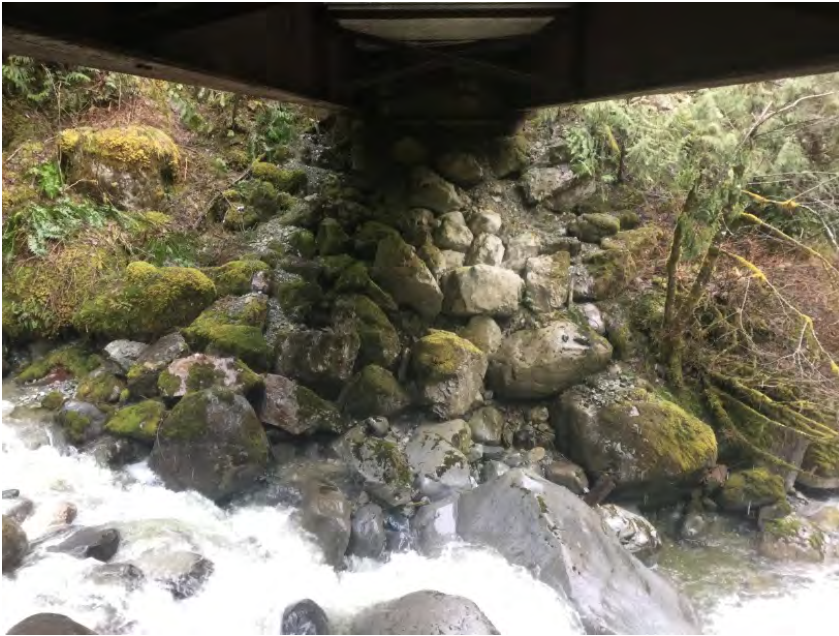
Left Bank Abutment when facing downstream
