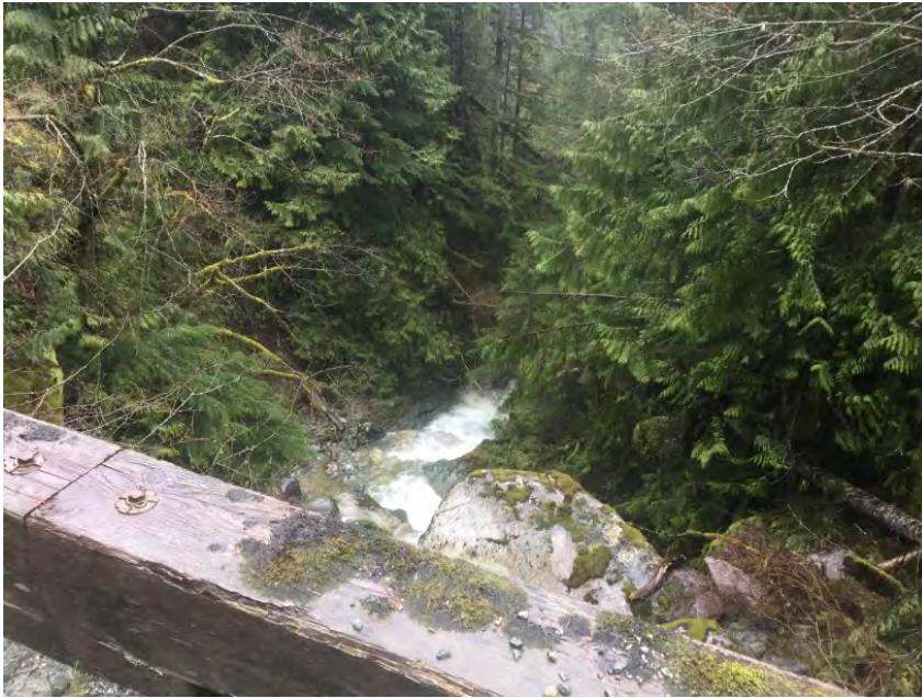
Looking downstream from deck
