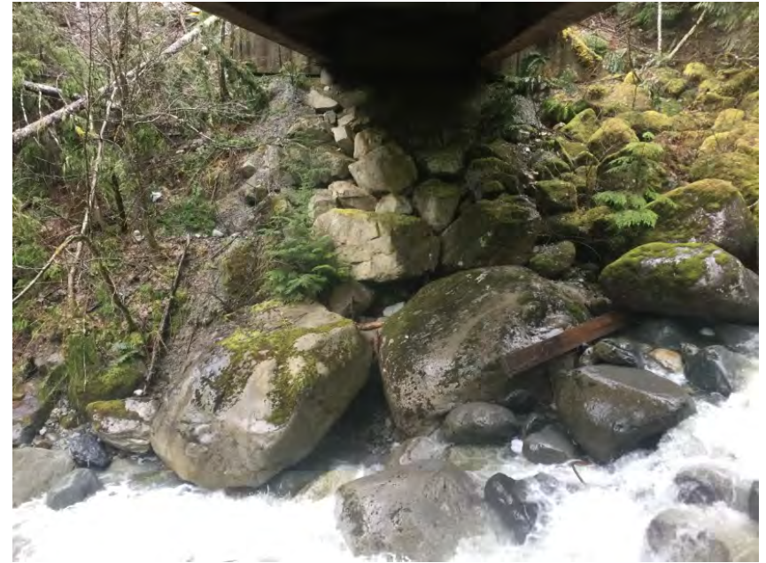
Right Bank Abutment when facing downstream
